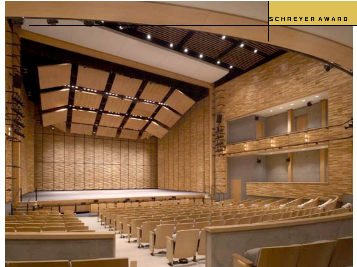
Above: view towards the stage with its carefully calibrated "acoustically transparent" canopy.
